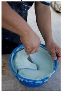
Follow manufacturer's instructions regarding water, mixing, slaking, and environmental conditions. Advanced thin-set mortars designed to be used only as instructed. Slaking simply means letting the mixed mortar sit, untouched, per the manufacturer's instructions. This is a key step that allows the chemical makeup of the mortar to work correctly. Not doing so, and using it immediately after the initial mix, will lead to the mortar getting stiff and quickly unworkable.
