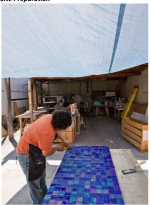
Transparent glass tile allows direct sunlight to pass through the tile and can significantly raise the temperature of the thin-set during the curing process. All areas to be tiled need to be shielded from wind and sun. Tile should be laid and cured in shade by using tarps, screens, or umbrellas.
